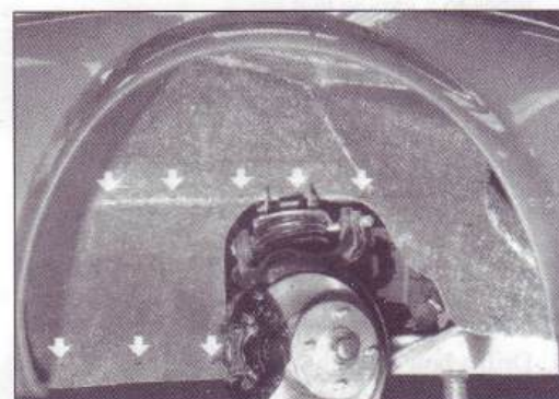
Fig.7d. Inner front wheel arch fitted showing rivet positions.
