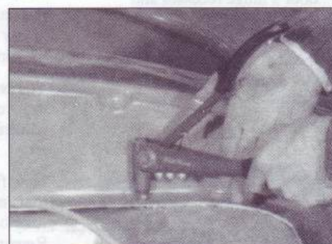
Fig.1d. Rivetting the front bulkhead to the chassis
