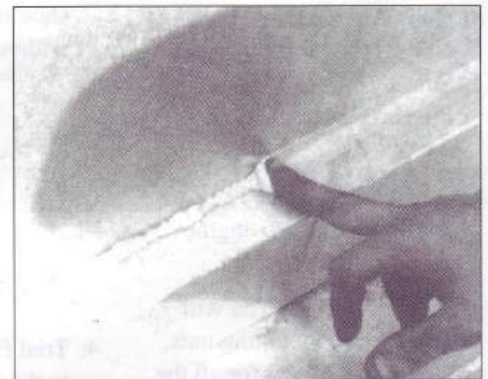
Fig.1b. Smoothing sealant to give a neat finish.
