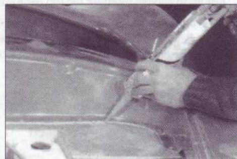
Fig.2d. Applying the sealant
